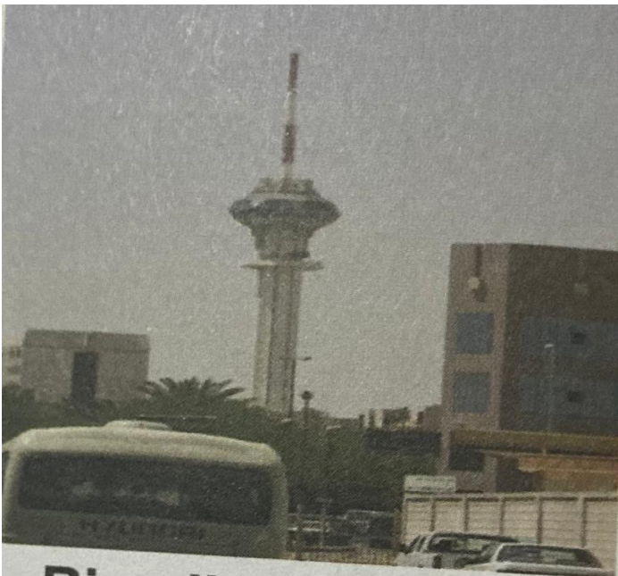
Riyadh TV Tower
